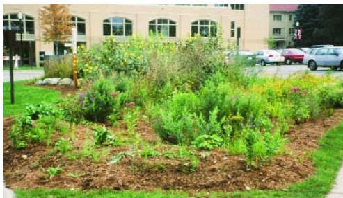
Bio Retention Area or Rain Garden in a Parking Lot
