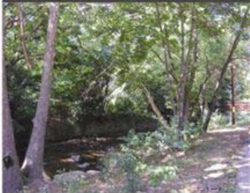
Parking lot near Central Avenue and Tookany Creek Parkway after the streambank restoration in 2003.
