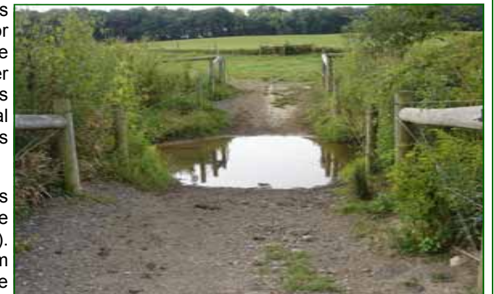
Above: Cement walkway continues across the stream to prevent animals from stirring up sediments in the stream while crossing.
