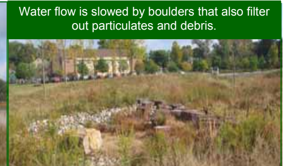
Water flow is slowed by boulders that also filter out particulates and debris. Stormwater moves through a swale, planted with grasses and sculpted to mimic a floodplain, which runs along Pennswood Village's entry road to an infiltration basin.
