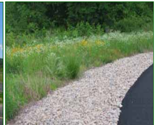
Above: View across a river stone bottom stormwater infiltration basin, surrounded by wet tolerant, native trees, shrubs, and meadow grasses. Below Left: View looking West into park from entrance off River Road. In the foreground is the river stone bottom of a stormwater infiltration basin planted with wet tolerant, native meadow grasses, trees, and shrubs. Below Right: River stone lined stormwater infiltration trench that parallels the edge of the park's driveway in key areas. Native meadow plantings are in the background along the woodland.
