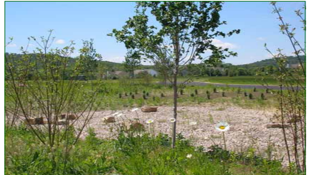
Above: View across a river stone bottom stormwater infiltration basin, surrounded by wet tolerant, native trees, shrubs, and meadow grasses. Below Left: View looking West into park from entrance off River Road. In the foreground is the river stone bottom of a stormwater infiltration basin planted with wet tolerant, native meadow grasses, trees, and shrubs. Below Right: River stone lined stormwater infiltration trench that parallels the edge of the park's driveway in key areas. Native meadow plantings are in the background along the woodland.
