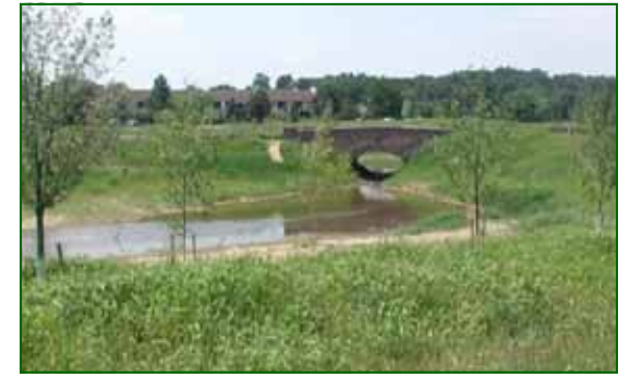
Above: Pond area after installation.
