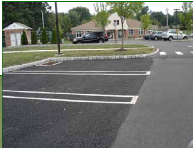
Above: Porous pavement shown at left and conventional pavement to the right in the parking facility at the Doylestown Commerce Center.
