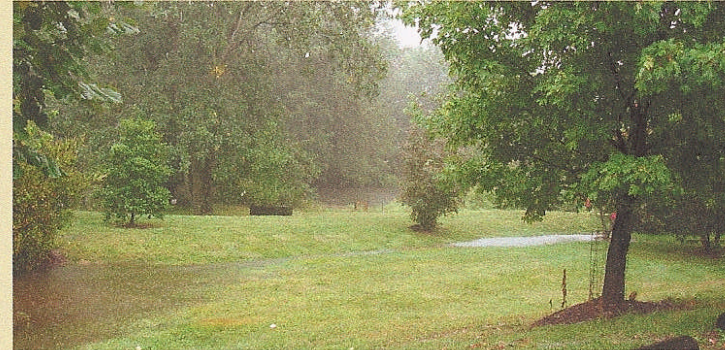
BEFORE: The traditionally designed detention basin had many shortcomings. The mowed grass did little to cool polluted runoff from the parking lot, and its shallow roots allowed minimal water to be absorbed into the soil. Sediment and pollutants quickly flowed through the basin and into the creek.
