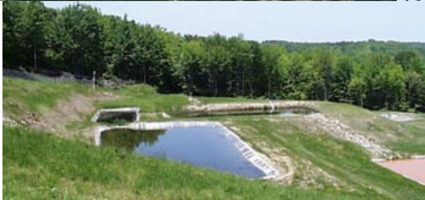
The water contaminated from the abandoned mine drainage is cleansed by flowing through a series of ponds and wetlands.
