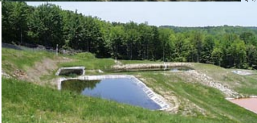
The water contaminated from the abandoned mine drainage is cleansed by flowing through a series of ponds and wetlands.
