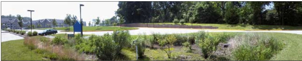
This traffic island on the Villanova University campus has a “bioinfiltration” system to capture water. Photo by Robert Traver.
